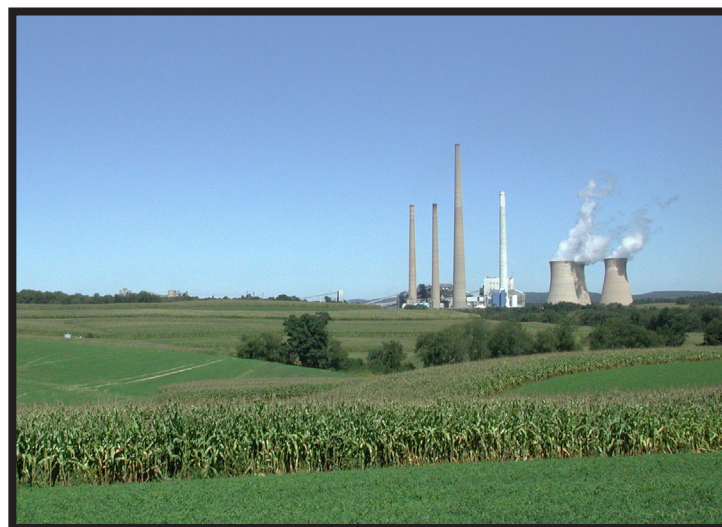
Homer City Generating Station, Homer City, PA
